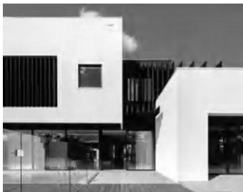
Exterior Wall Cladding
